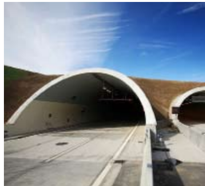
Two tunnels that are 2 km (1.2 mi.) long are part of the ring road around Prague, Czech Republic.
