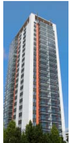
Rising above Espoo outside Helsinki, Finland, is the 70 m (230 ft.) Leppävaara tower with its 113 apartments. Residents of the 21-story building have access to a common sauna department and a roof top terrace.
