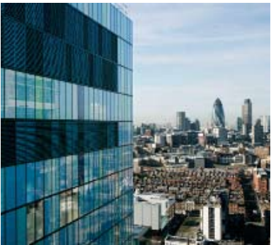
Two London hospitals, Barts and the London Hospital, are part of one project worth GBP 1 billion. The London Hospital in Whitechapel (above) will be the largest hospital in the U.K. The general public in East London will have access to both general and specialist care, along with emergency and pediatric wards.
