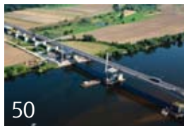
50 Phase II of the A1 expressway, Poland
