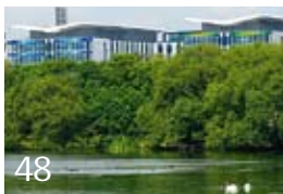
48 Europe's largest geothermal lake loop in Nottinghamshire, U.K.
