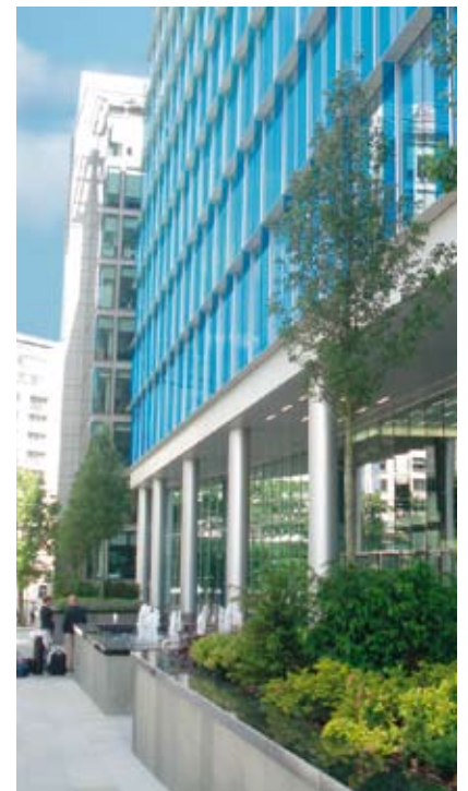
One Kingdom Street at Paddington-Central in London utilizes both geothermal heat and solar panels to reduce its climate impact.
