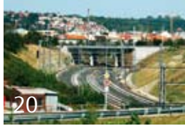
20 New railroad hub in Prague, Czech Republic
