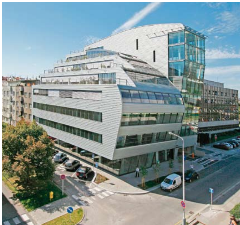
Vyšehrad Victoria is Skanska's latest commercial development project in Prague, Czech Republic. An architecturally distinctive project with 4,750 sq. m (51,000 sq. ft.) of office space. It offers green walk-on terraces as an extra amenity for tenants.
