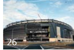
26 New technology for more efficient stadium construction
