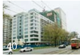
40 The Skanska street in Warsaw is growing
